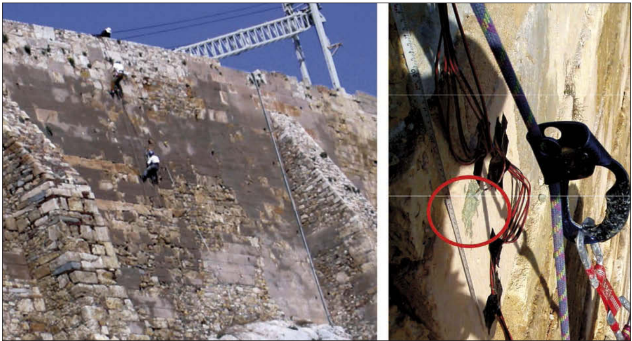
Fig. 2. Climbers fitting the cable on the wall (left), bentonite electrode (right).
