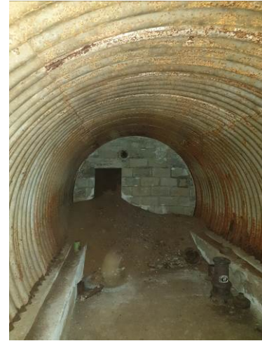
Figure 3: Photograph of WW2 underground Operational Base in Suffolk, UK)
